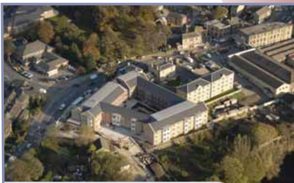
Aerial view of Royd Court under construction
